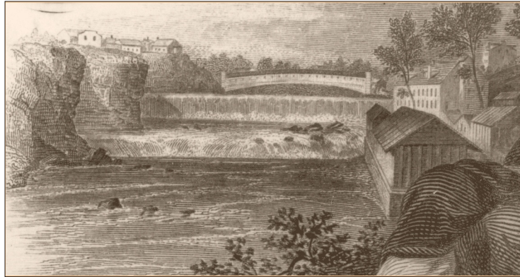
Post 1837 images of the Barclay dam and the record-length 262 foot Burr Arch bridge at Saugerties.
